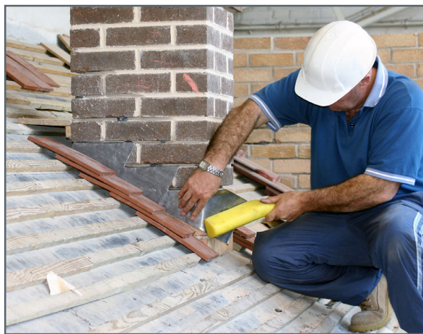
Figure 4.4. Installation of roof curb around a chimney.
