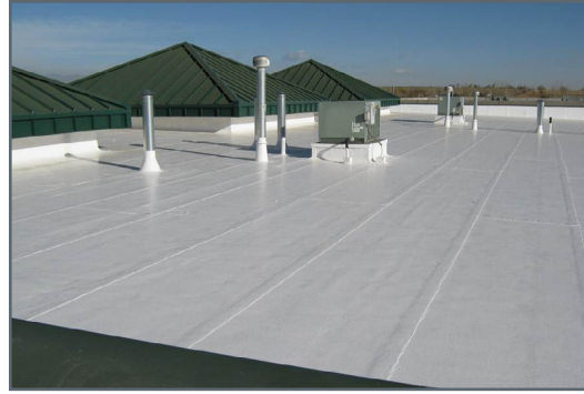
Figure 4.1. Top: highly reflective white flat roof 4 ; bottom left: low-slope metal roof; and bottom right: shingle roof.
