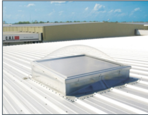
Figure 4.3. Left: installation of skylight on roof; right: installed roof dome skylight with flashing (Photos courtesy of DayStar).
