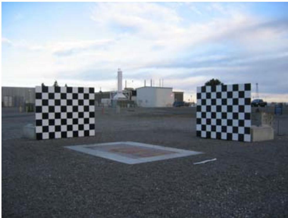
Drop Pad Area Looking Northwest
