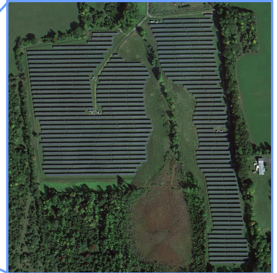
4.8 MW Grand Isle solar farm, connected at end of 12.47 kV distribution feeder
