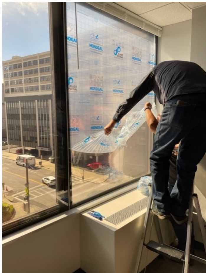
Figure 1. Commercial secondary windows are far easier and less expensive to install compared to full window replacement. (Photo courtesy of Intelligent Energy Group)
