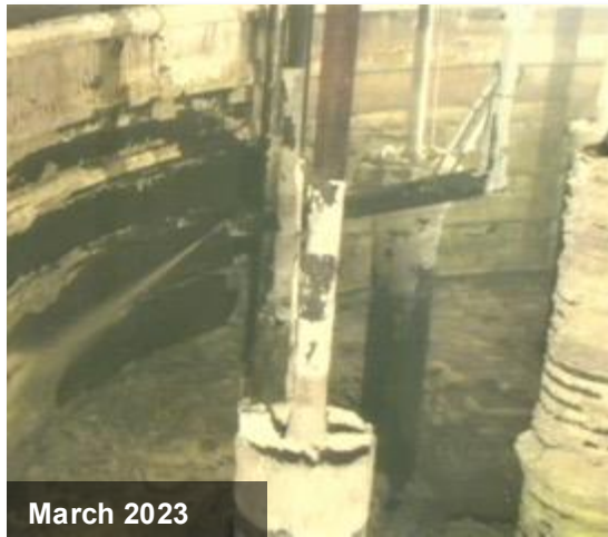
Modified sluicing inside Tank AX-101
