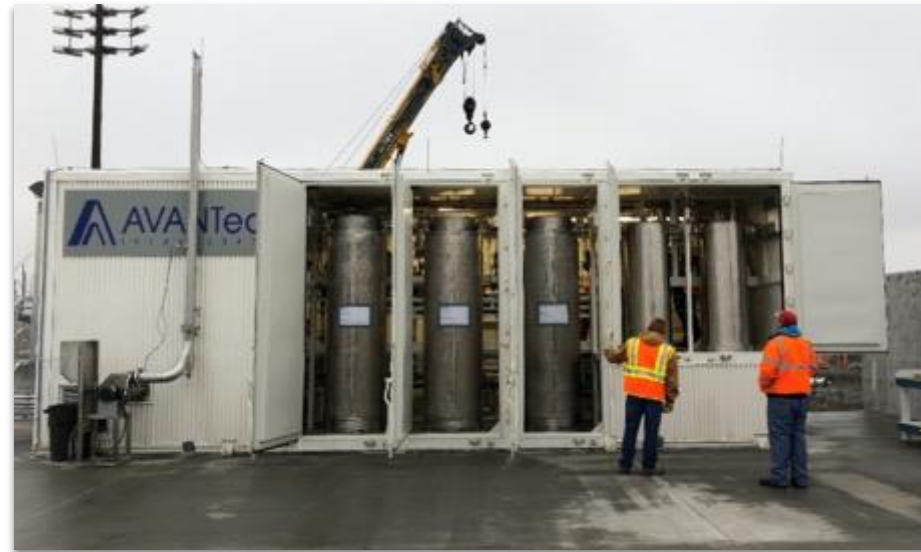
TSCR unit showing ion exchange and filter units
