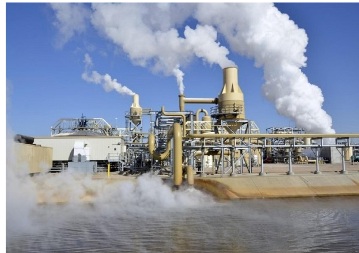
Geothermal power plant near California's Salton Sea
