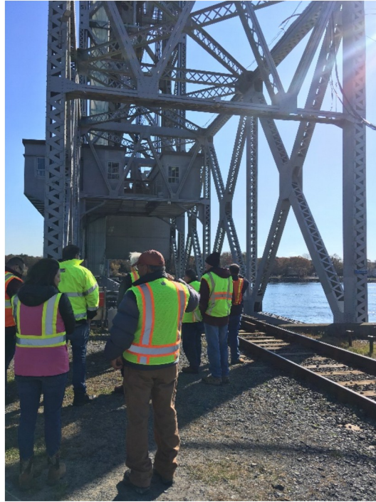
Fig. 3. Examining the condition of the Cape Cod Canal Bridge
