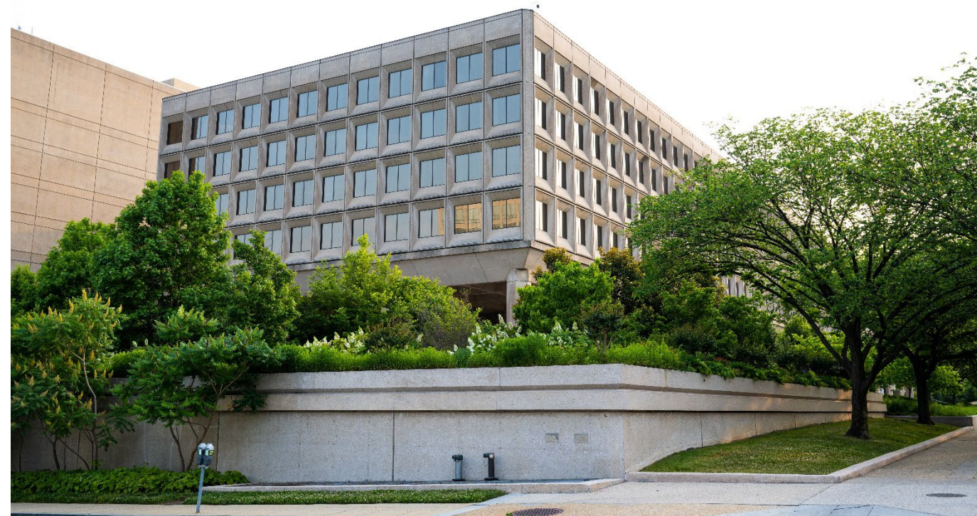
Forrestal Building, Washington, D.C.
