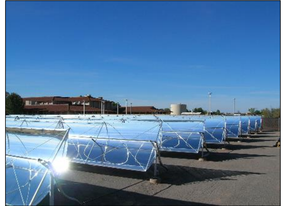
Solar panels supply energy to operate the groundwater-treatment plant
