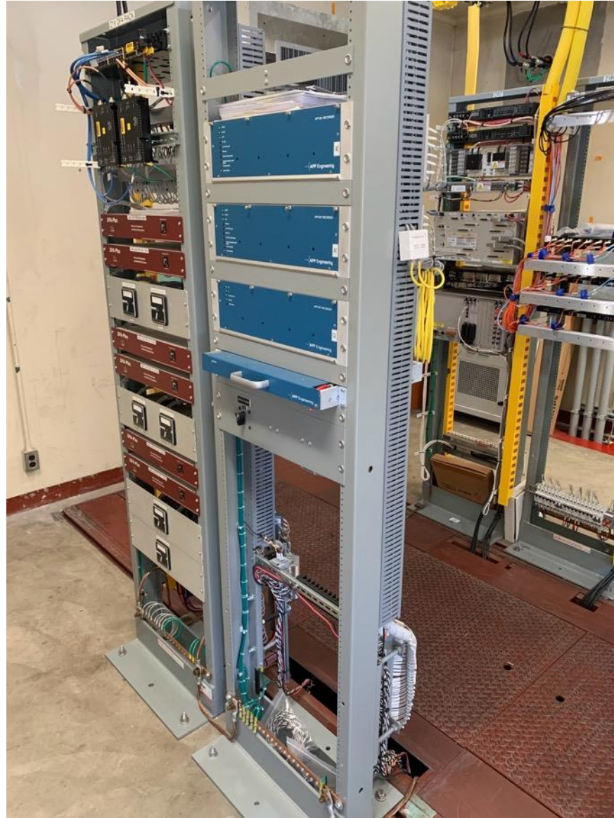
Digital fault recorder at a distribution substation Photo courtesy of Southern California Edison
