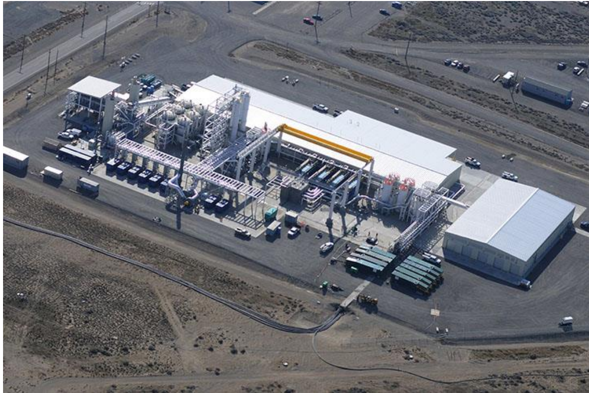
200W P&T Facility
