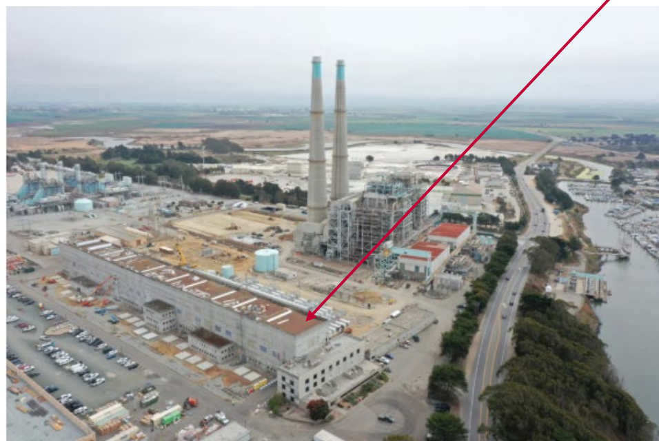
Aerial view of the site taken in 2020: the long building in the foreground is a former turbine hall which housed MOSS300. Image: LG Energy Solution
