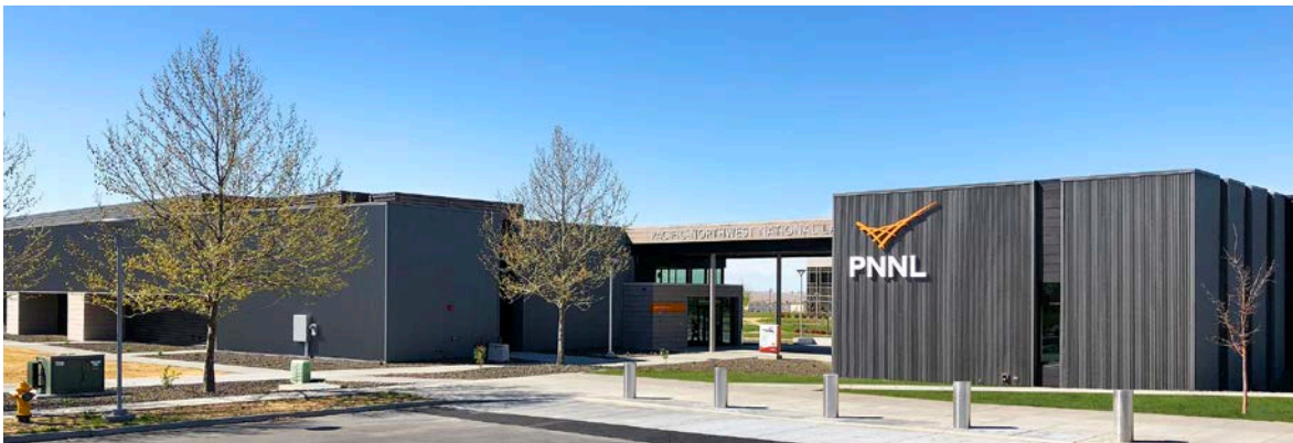
Figure 4. PNNL’s New Discovery Hall Building in Richland, Washington
