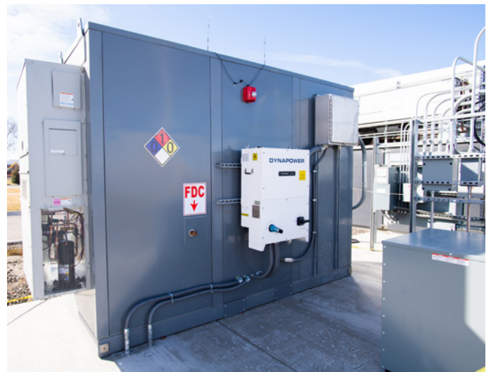
The 125 kilowatt (kW), 250 kW-hour lithium-ion battery at PNNL will make it possible to explore new aspects of grid services and use of clean energy.
