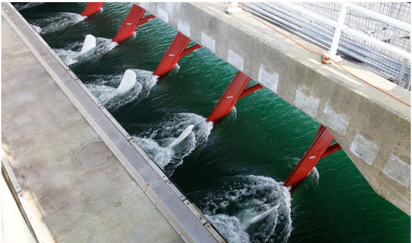
Tidal turbines at the 1.25 MW Oosterschelde Tidal Power Plant in the Netherlands.
