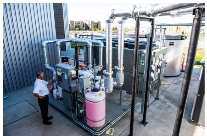
The thermal energy storage system, adjacent to PNNL's Systems Engineering Building, includes a pumping station (foreground), chiller unit (middle), and three large ice storage canisters.
