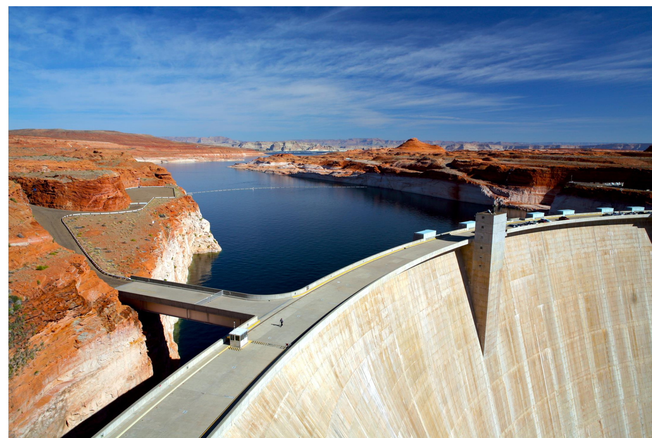
Pictured here is the Glen Canyon Dam, which provides power to multiple states in the western United States. It has been significantly impacted by ongoing drought conditions in the region. Dynamic models, such as the ones being developed in this project, will support better hydropower modeling that takes into account extremes in water conditions to support better planning for the future. (Photo by Dauf | Shutterstock.com)
