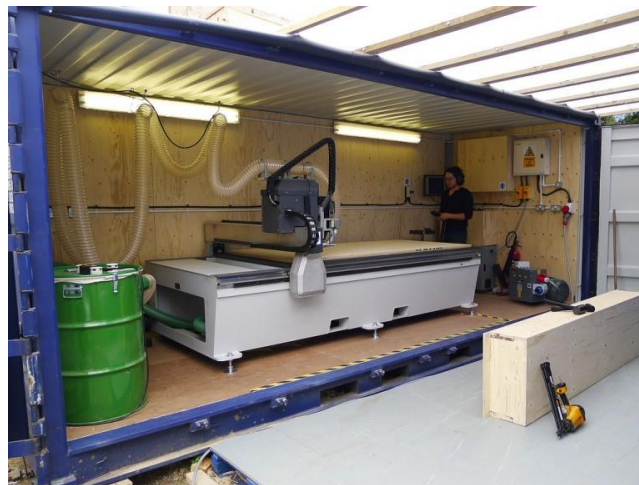
Figure 7. Facit's CNC machine, transported to home sites in a shipping container, cuts customized pieces for homes. (Source: Facit)
