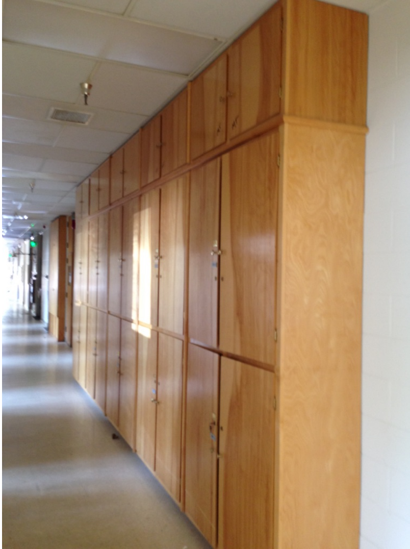
Figure 10. Original Hallway Cabinets and Doors in Building 520
