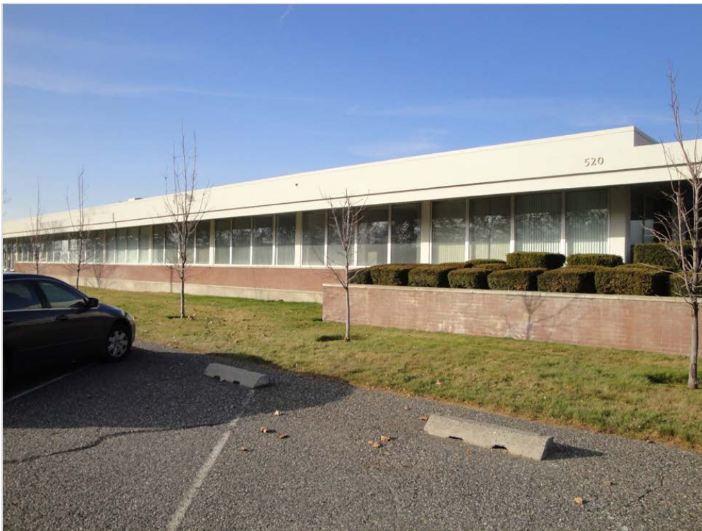
Figure 2. RTL 520 South (Front) Elevation (Harvey et al. 2015)
