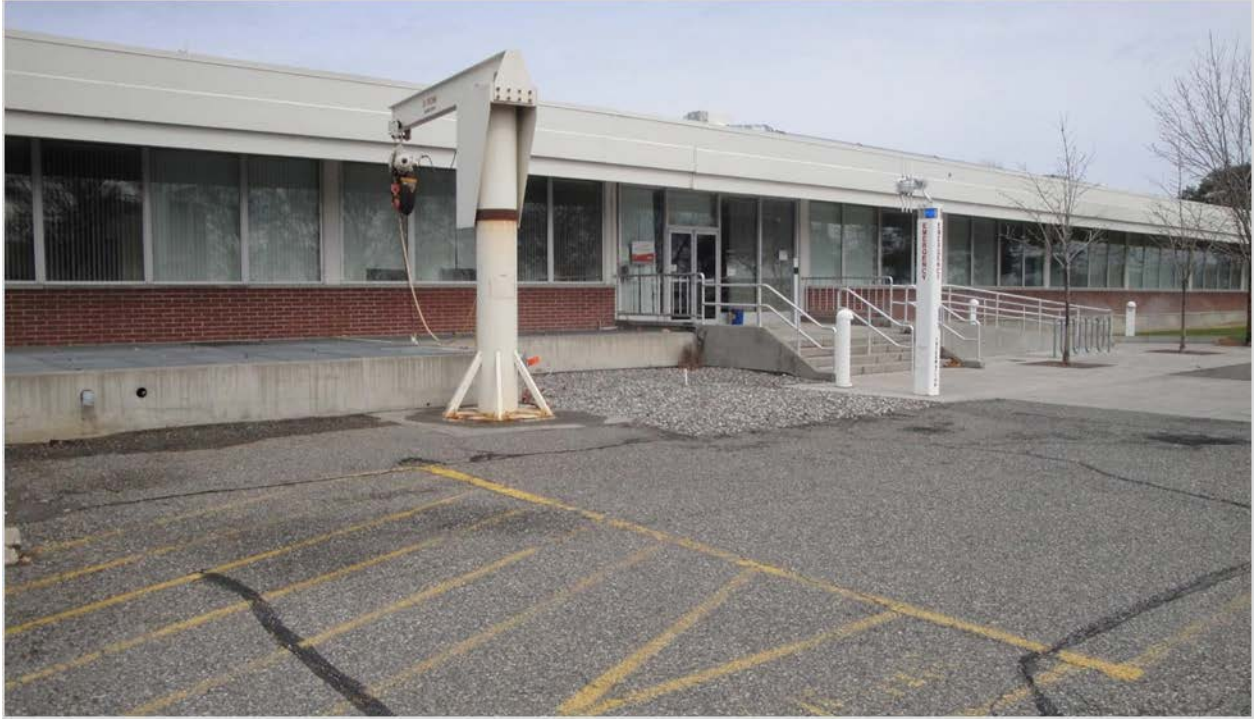
Figure 3. RTL 520 South (Front) Elevation (Harvey et al. 2015)
