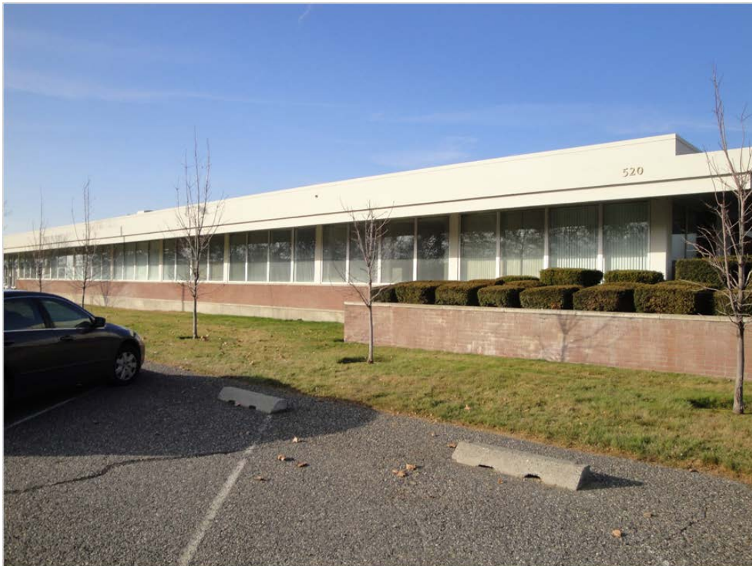
Figure 2. RTL 520 South (Front) Elevation (Harvey et al. 2015)
