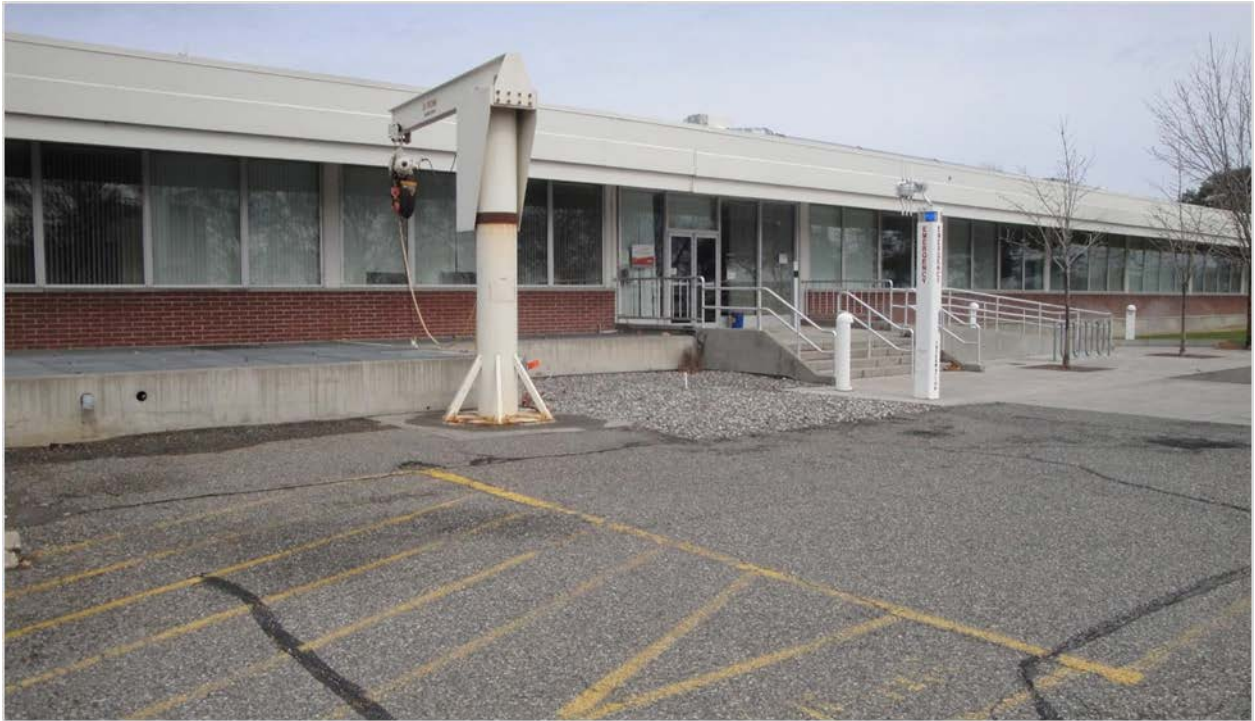
Figure 3. RTL 520 South (Front) Elevation (Harvey et al. 2015)
