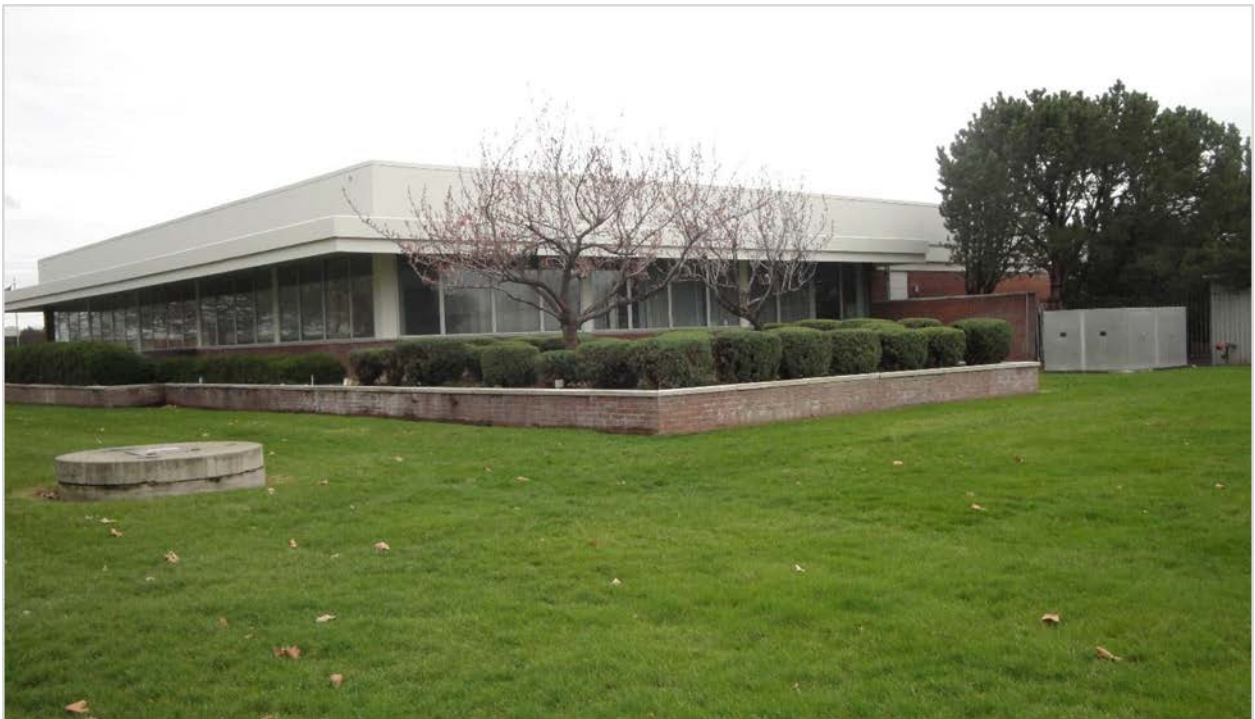
Figure 4. RTL 520 Northwest Corner (Harvey et al. 2015)
