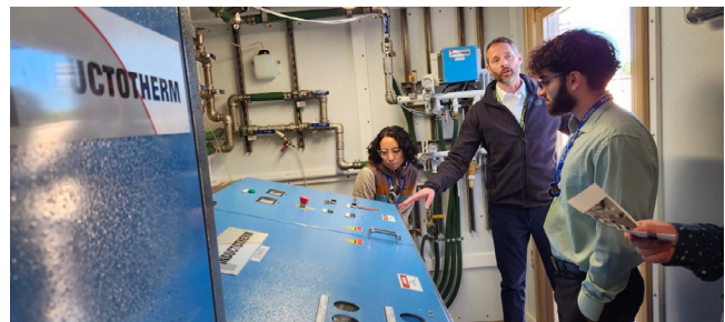
Photo by Pacific Northwest National Laboratory
