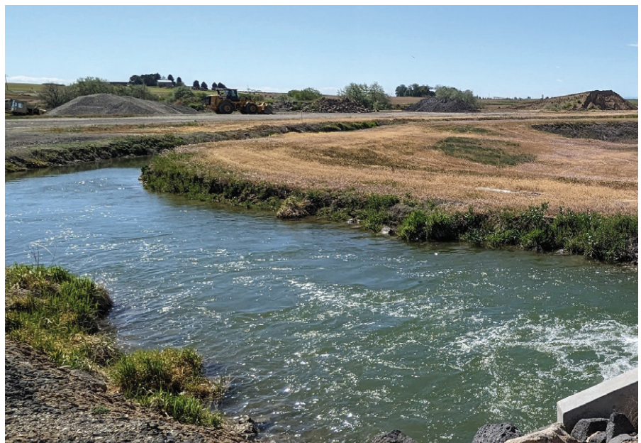
Earthen canal, North Side Canal Company, Jerome, Idaho. Photo by Jed Jorgensen.
