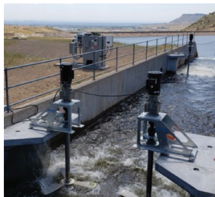
Hydrokinetic turbines deployed in canals. Photo credit: Emrgy
