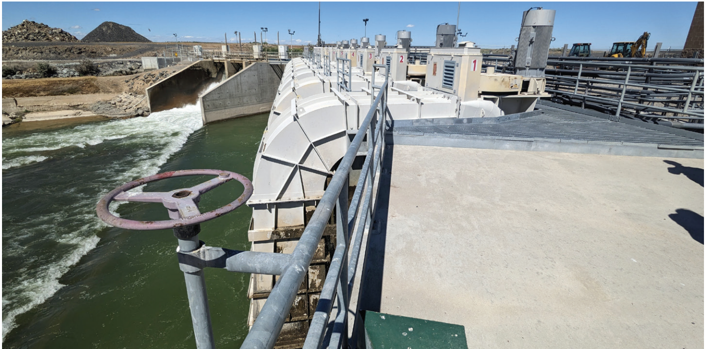
Drop structure hydropower installation with eight Mavel siphon turbines. North Side Canal Company, Jerome, Idaho. Photo by Jed Jorgensen.
