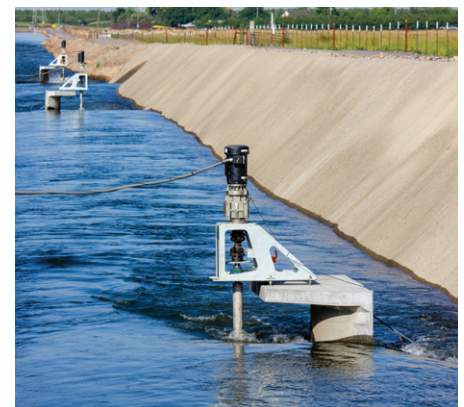
Drop structure hydropower installation with eight Mavel siphon turbines. North Side Canal Company, Jerome, Idaho. Photo by Jed Jorgensen.
