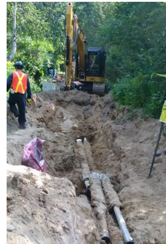
Chalk River Laboratories Site - Remediation of Pipeline
