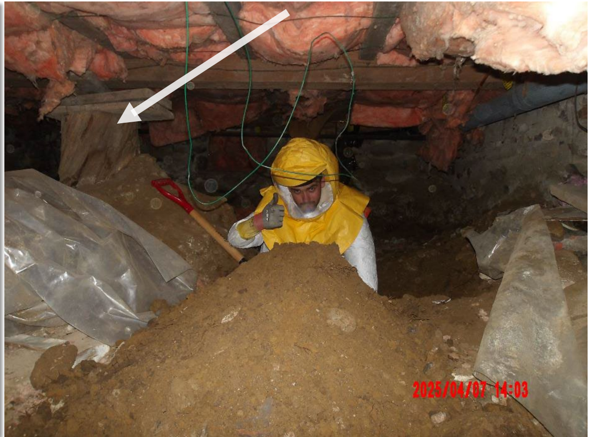
Tree stump used as part of main structural support
