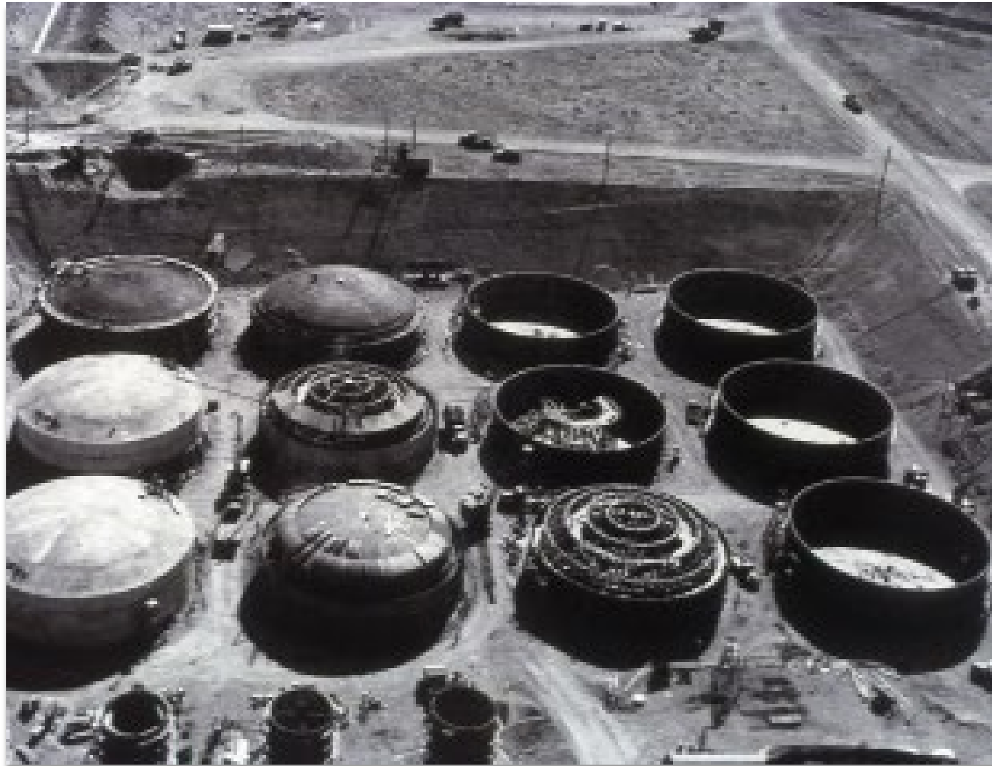
Construction of large underground waste tanks.
