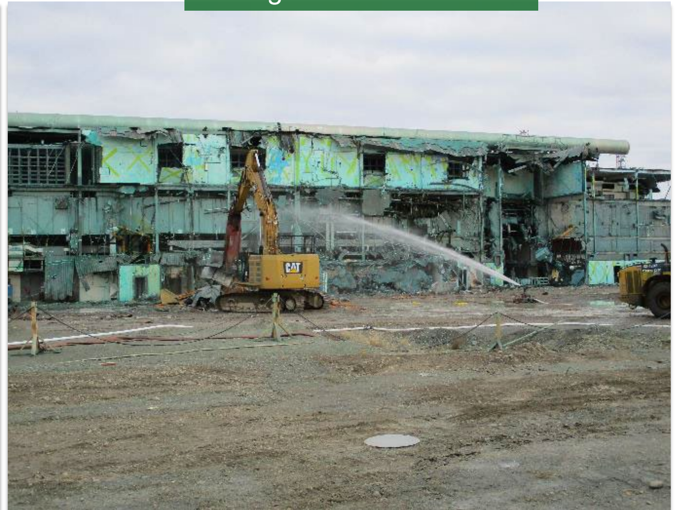
Demolition of the main Plutonium Production Facility.
