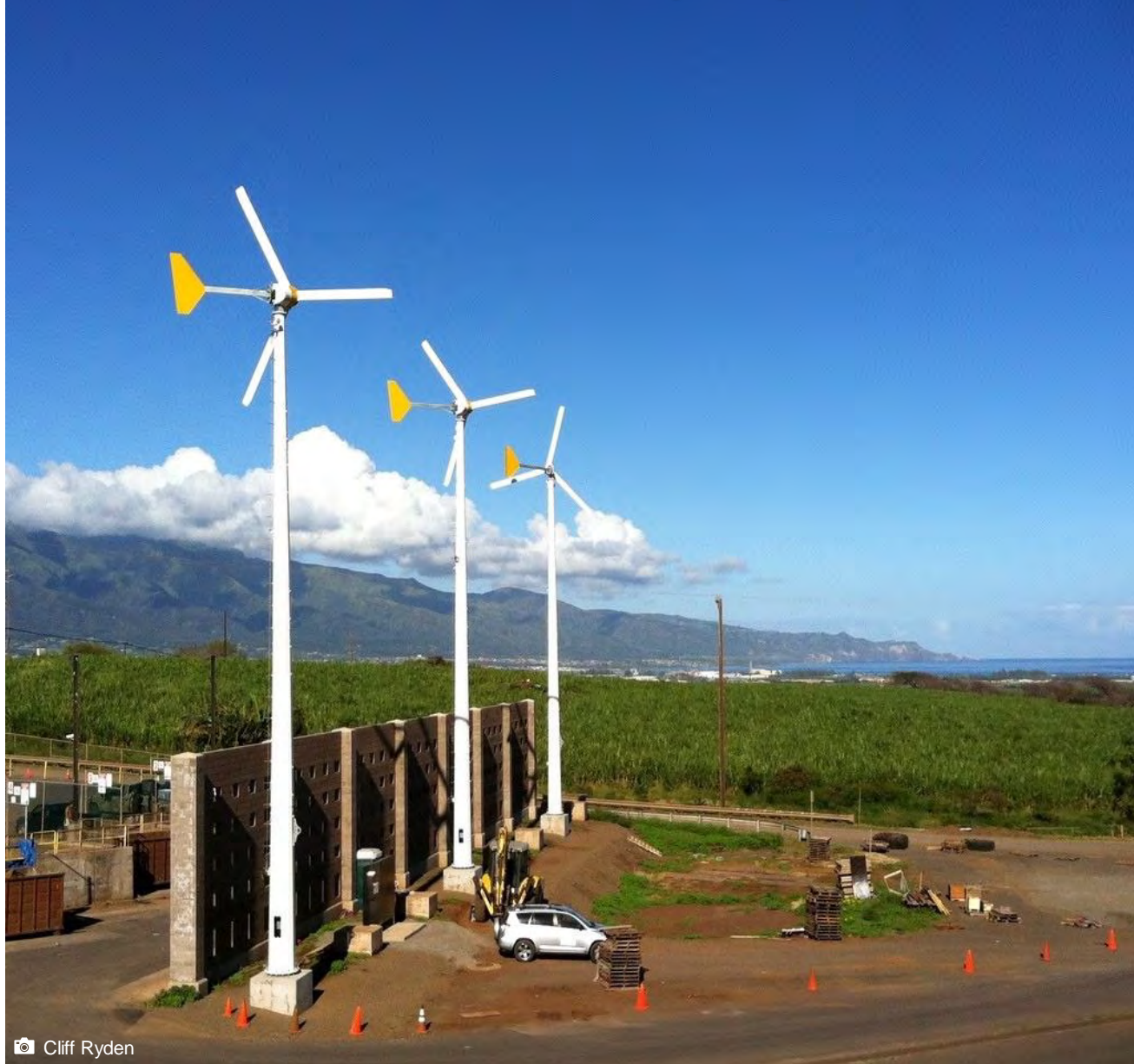
Central Maui Landfill and Recycling Center, Hawaii
