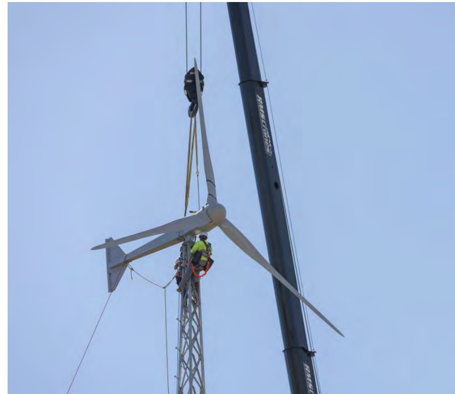
Construction crews install a 15.6 kW wind turbine (Photo: Joe DeINero, NREL)
