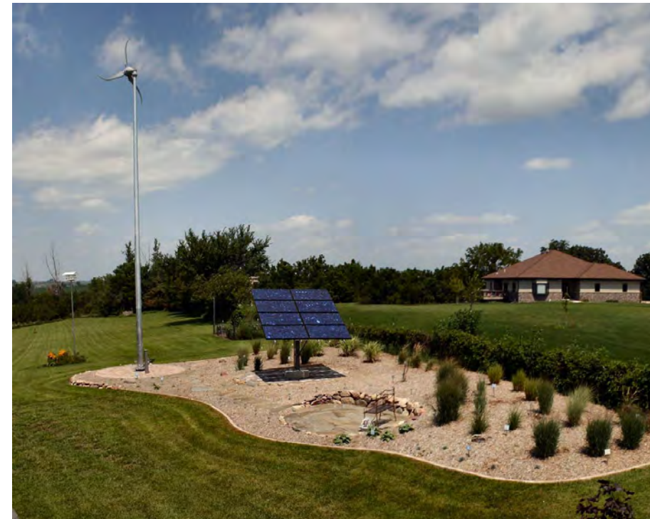
A small hybrid system with a wind turbine and solar panels (Photo: Todd Hannen)
