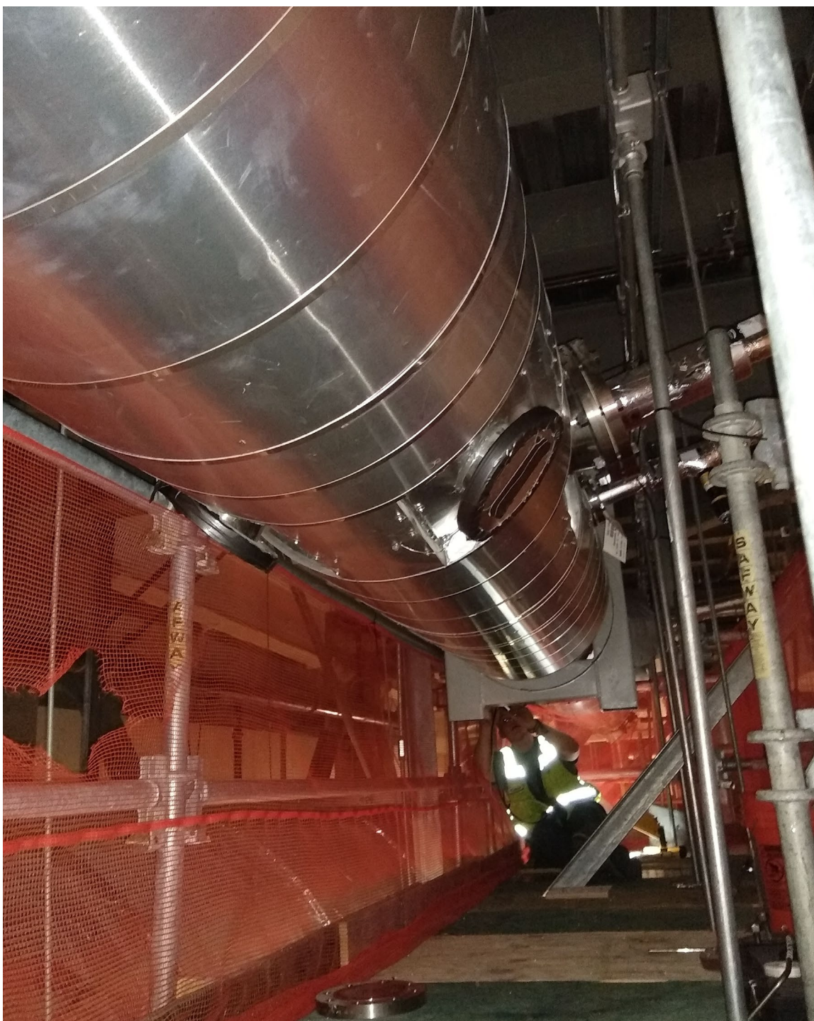
Figure 4. LAW LV-S3 Stack. The pair of ports to characterize the record sampler port location is visible in the foreground (near the center of the image) while the ports to characterize the CAM is in the background, at the location of the Bison staff member. The stack is positioned near the center of the L-0320 Stack Monitoring Room, and the photograph is nominally pointed to the north. Stack flow is from the foreground (south) to background (north).
