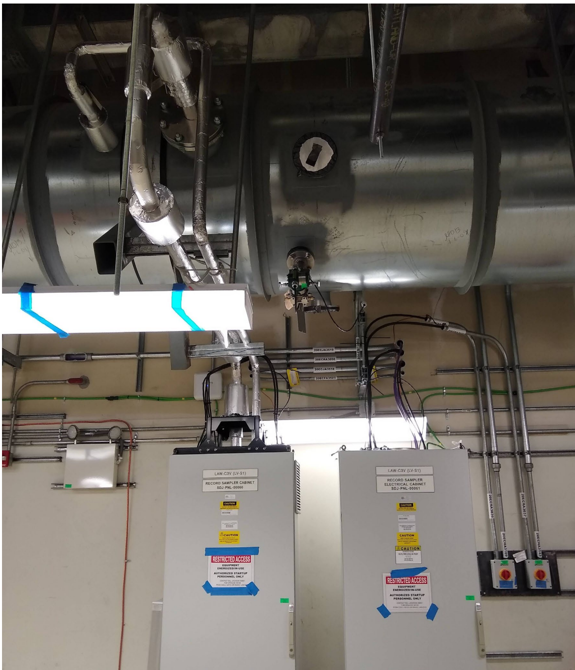
Figure 2. LAW LV-S1 Stack. The stack is positioned along the west wall of the L-0320 Stack Monitoring Room, with one test port slightly below the horizontal centerline, and the second test port slightly west of plumb (behind the probe in the photo). Stack flow is from left (south) to right (north).
