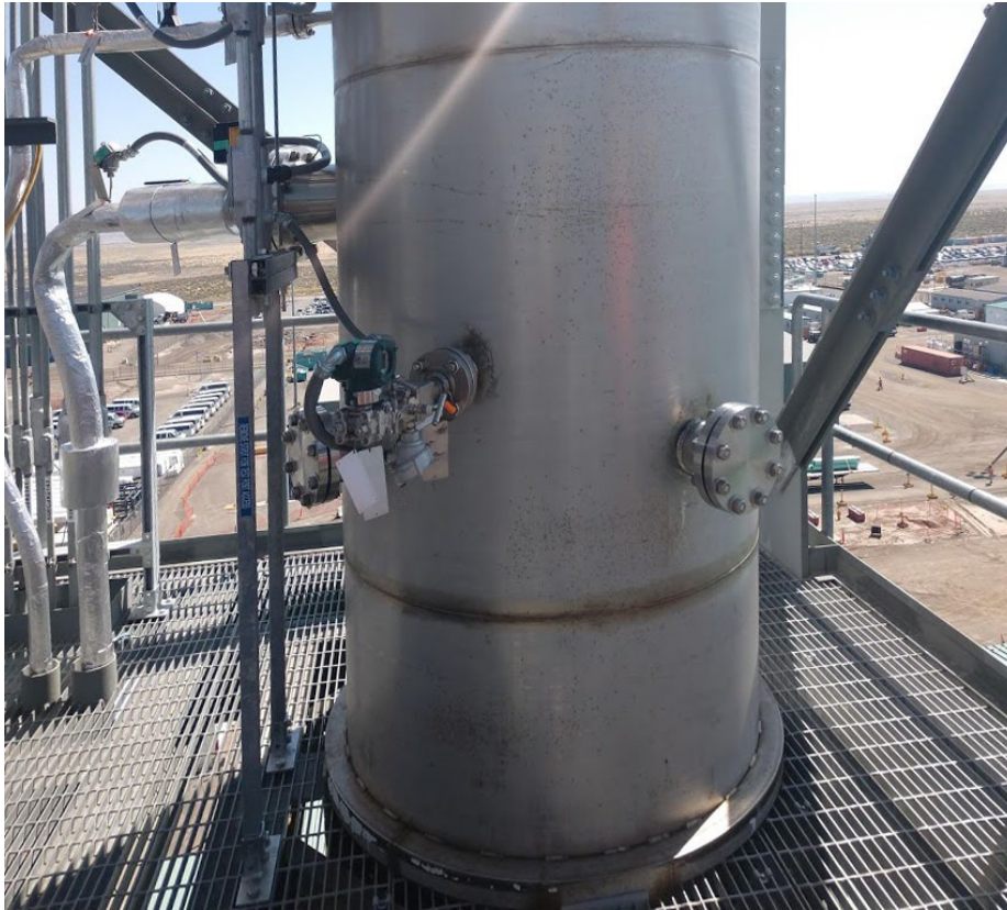
Figure 1. LAB LB-C2 Stack. In this photograph, each port is covered with a large plate secured by eight bolts. The stack flow meter is visible as the large collection of equipment located slightly left of stack center in this photograph.
