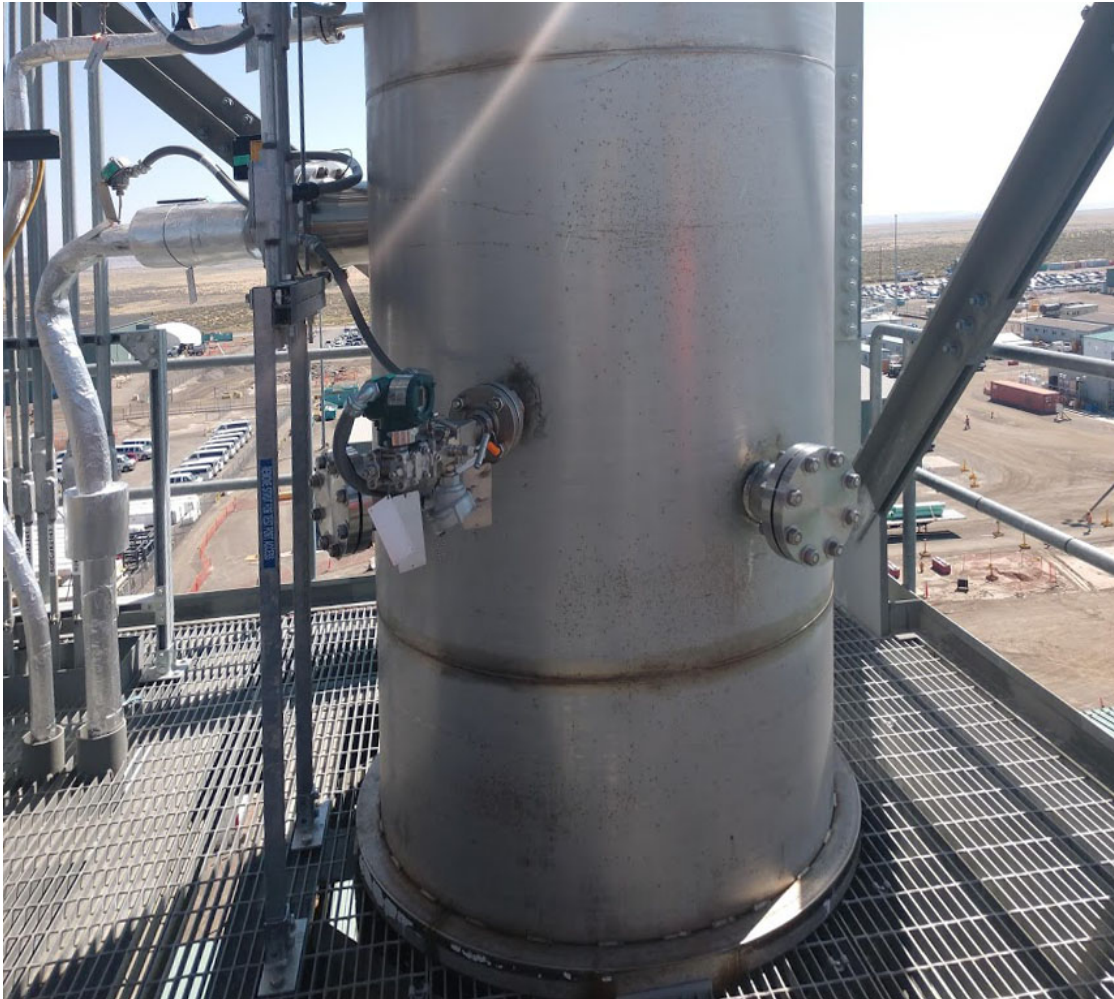
Figure 1. LAB LB-C2 Stack. Each port is covered in this photo with a large plate secured by eight bolts. The stack flow meter is visible as the large collection of equipment located slightly left of stack center in this photograph.
