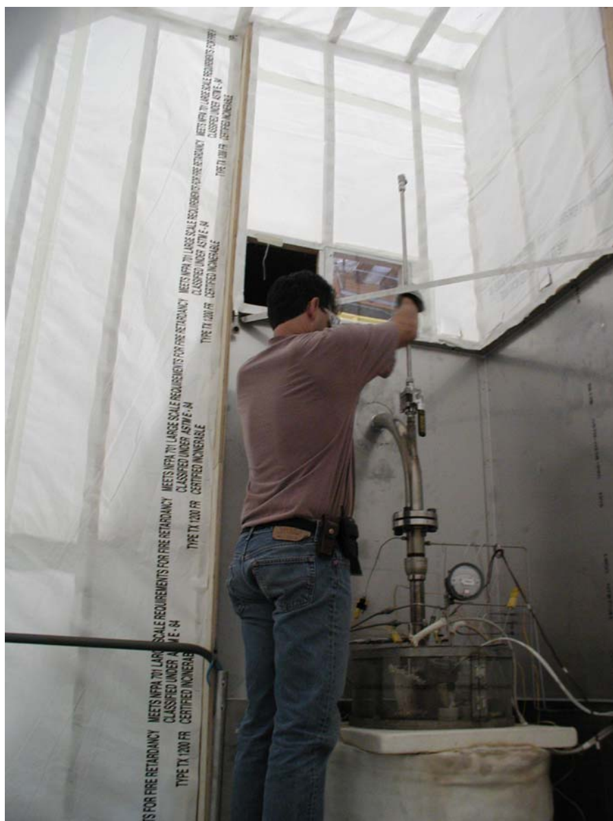
Figure 4.14. Melter Off-Gas Line Sampling Port
