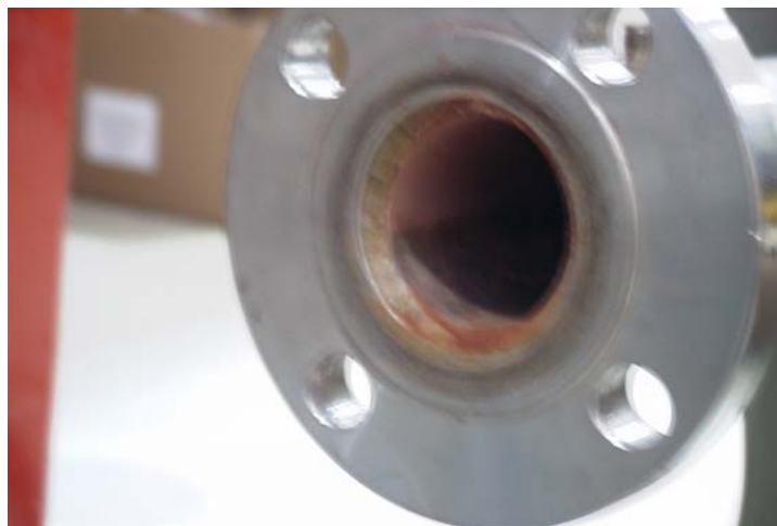
Outlet of Horizontal Pipe Section, View E
