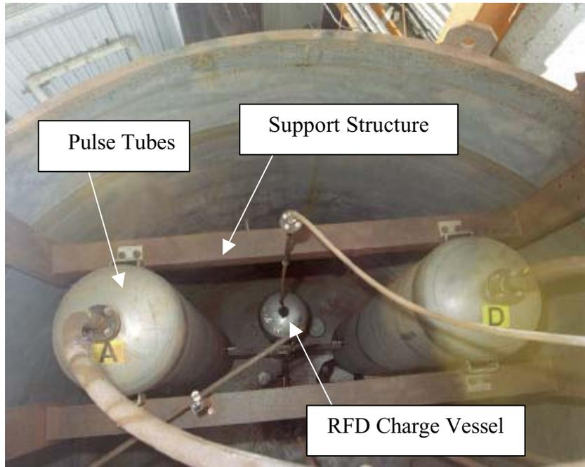
Figure 2.6. Photograph of Two Pulse Tubes and the RFD Charge Vessel Installed in the Tank.
