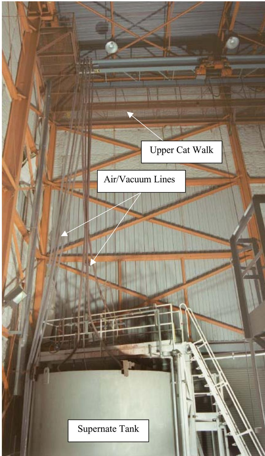
Figure 2.7. Photograph showing the Air/Vacuum Lines to the Pulse Tubes
