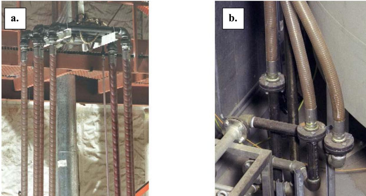
Figure 3.9. Photographs of the Air/Vacuum Lines Showing Slurry Coating at (a) Top of the Upper Cat Walk and (b) Control Module.
