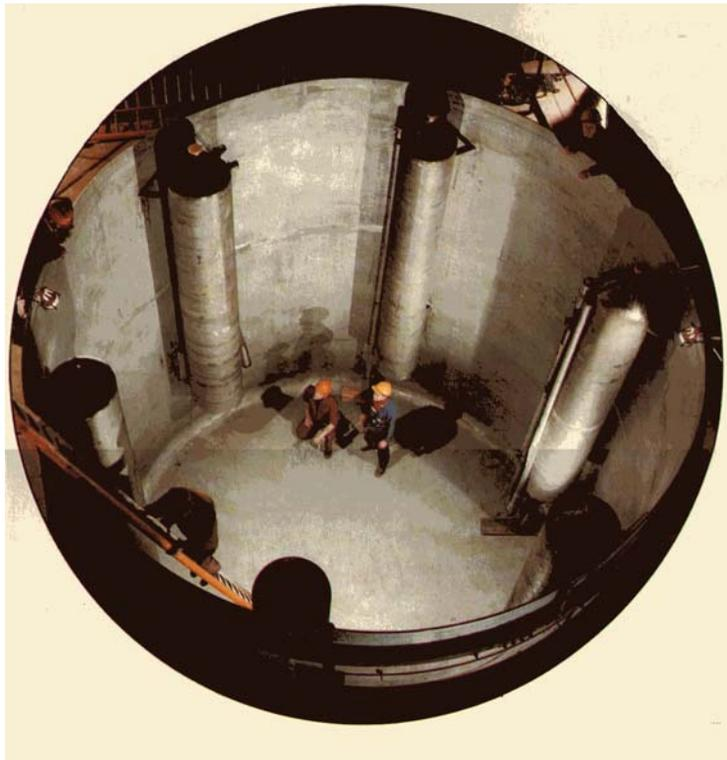
Figure 1.2. Pulsed Jet Mixers in BNFL's Highly Active Liquid Storage Tanks
