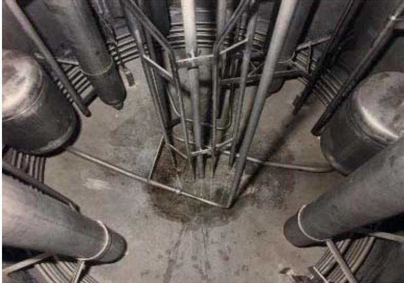
Figure 1.1. Pulsed Jet Mixers and RFD's Installed in BNFL's Encapsulation Plant in Sellafield, UK.
