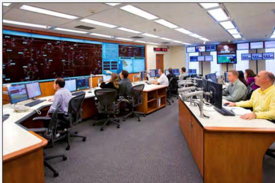
Building upon expertise in electricity transmission and distribution, PNNL created the Electricity Infrastructure Operations Center, a functioning control room that brings together industry software, real-time grid data and advanced computation. Shaped with input from utilities and researchers across the Northwest, technologies developed and tested here can be transferred to industry and address the national need to better manage and control the grid.
