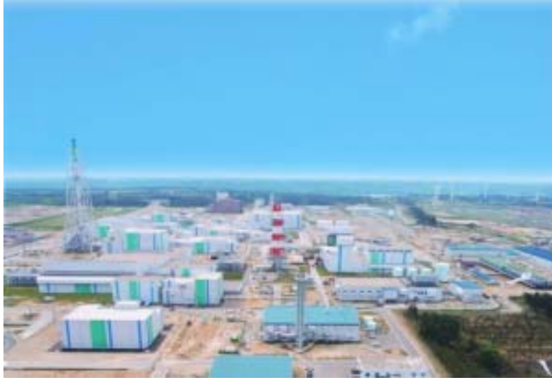
Figure 1: Rokkashomura Reprocessing Plant (RRP) Complex
