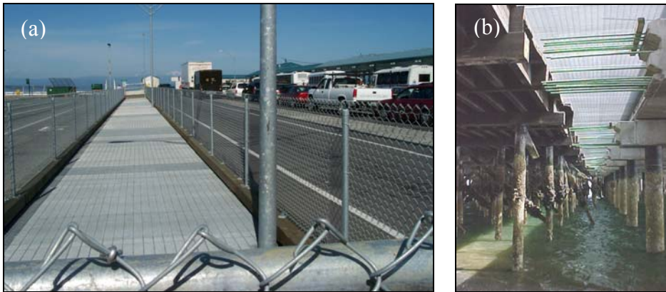
Figure 8. Deck grating from above (a) and below (b) (note the sun/shade pattern on the water surface).
