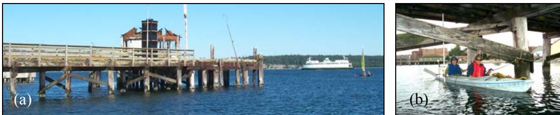
Figure 7. (a) Sun Tunnel installed at the existing dock in Port Townsend, Washington; (b) Measuring light under the dock.
