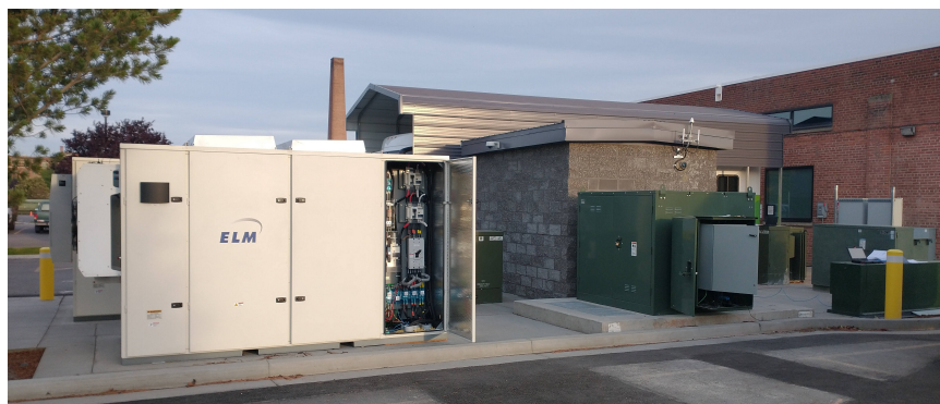
Figure 23. 500-kW BESS and microgrid control shed behind CCRS, August 10, 2021.
