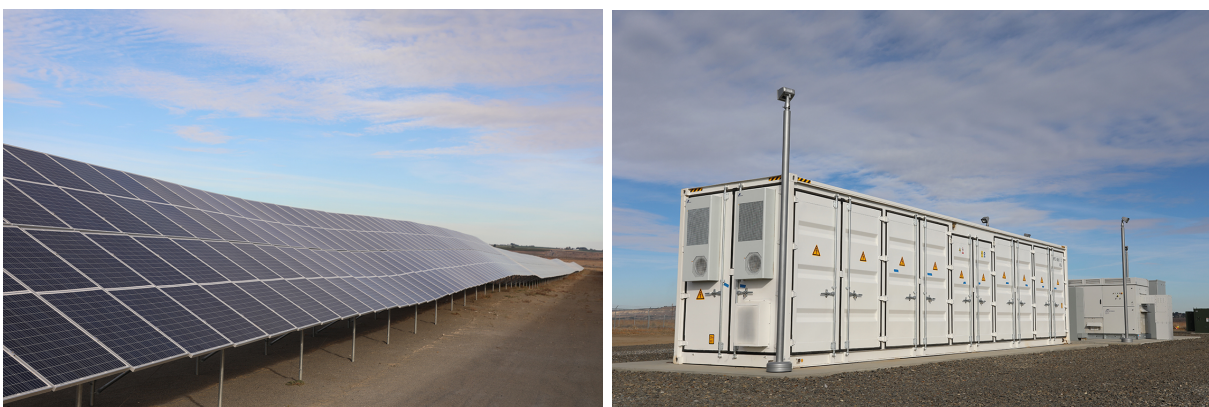
Figure 1.2. Large-scale PV and BESS at Horn Rapids.
