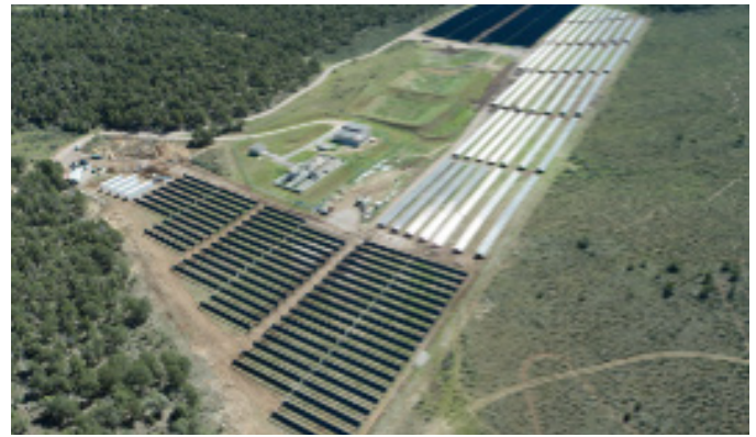
Figure 2. Solar panels and battery energy storage systems at Colorado Mountain College's Spring Valley Campus. 4
