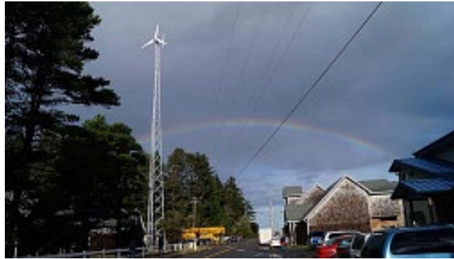
Figure 71: University of Oregon 10 kW Wind Turbine 1
