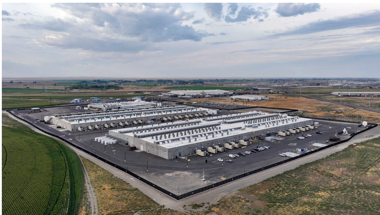
Figure 30: Amazon Web Services Data Center, Boardman Oregon, 2024 4
