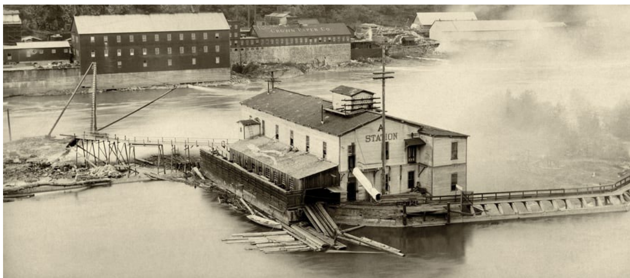
Figure 8: Willamette Falls Powerhouse and Oregon's first High-Voltage Transmission Line 1
