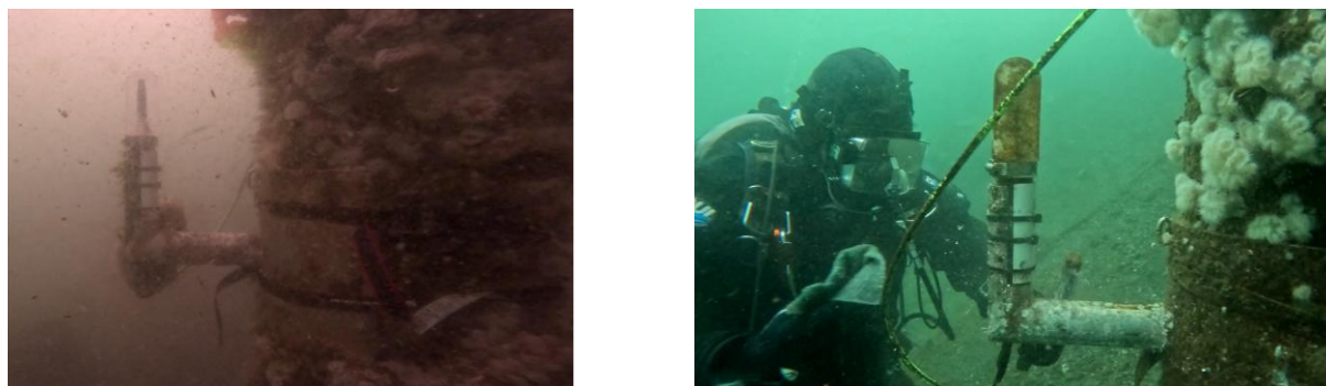
Figure 7: Pier-mounted hydrophone with flow shield upon deployment (August 2025) and during diver inspection (March 2026).
