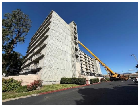
Figure 1. Crane for lifting the CHPWH Equipment onto Casa Panorama roof
