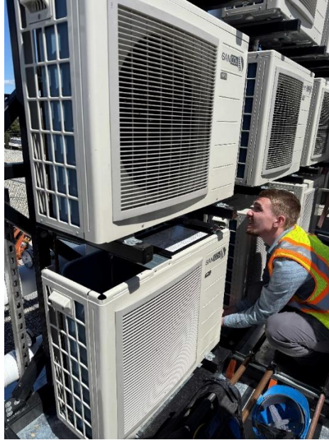
Figure 2. Mechanical Engineer inspecting the front of the Droplet-9 at Casa Panorama
