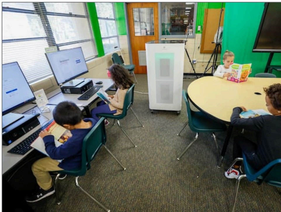
PAC classroom installation at Dekalb School District, Atlanta, GA
