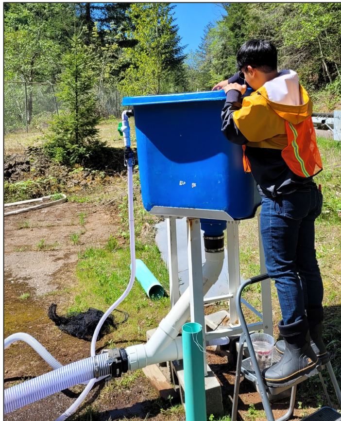
Figure 3-2. The control release system at GPR. The hose on the left near the top of the blue release tank supplies flow-through water to the basin. Water is also supplied to the PVC Y-piece to provide constant flow through the release hose.
