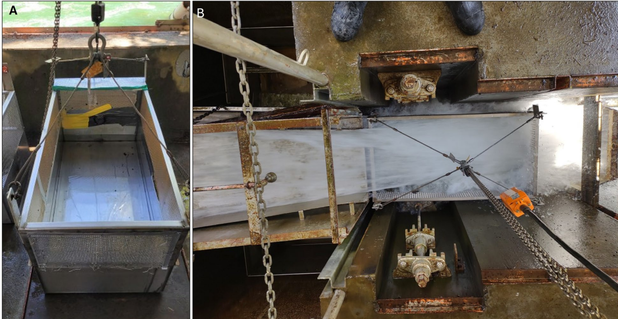
Figure 3-1. Multiple views of the juvenile collection basket at Green Peter. (A) A view of the juvenile collection basket out of water. (B) An aerial view of the juvenile fish collection basket in water, with the juvenile bypass pipe on the left flowing into the basket. The water is flowing out of the basket into the tailwaters on the right side of the picture.
