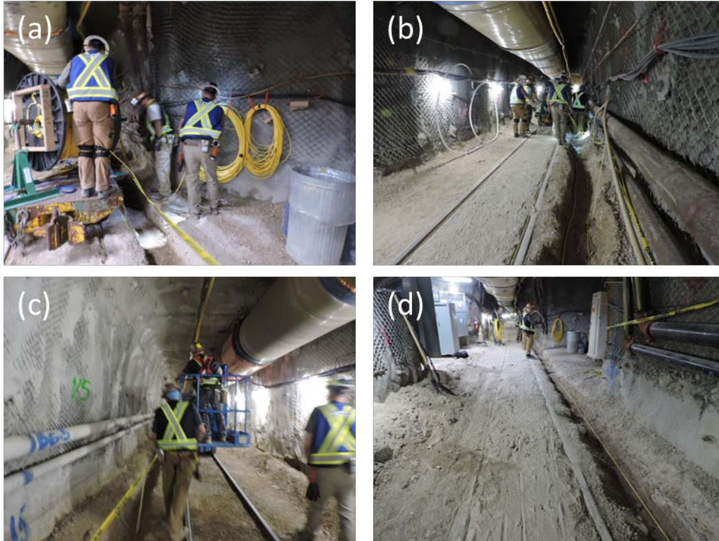
Figure 6. Photographs of the emplacement in the .06 Bypass drifts showing (a) cable reels on rail cars, (b) staff pulling the cable off the reel, (c) guiding the cable into the trench, and (d) the final placement of the cable in the trench. Photos by K. Chojnicki.
