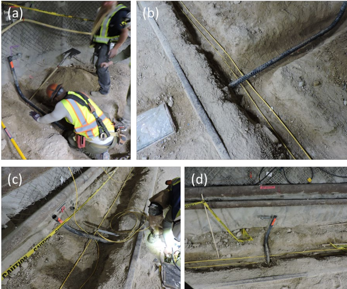
Figure 7. Photographs showing an example of cables being routed around existing infrastructure in the tunnel by (a) digging a trench below this pre-existing cable conduit, and then (b, c, d) routing the cable under the conduit(s). Photos by K. Chojnicki.
