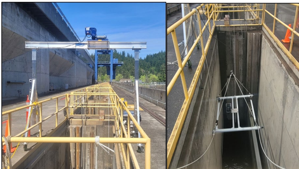
Figure 2.4. Imaging sonar deployment system. Portable deployment gantry (left) and submerged sonar mounting platform (right).
