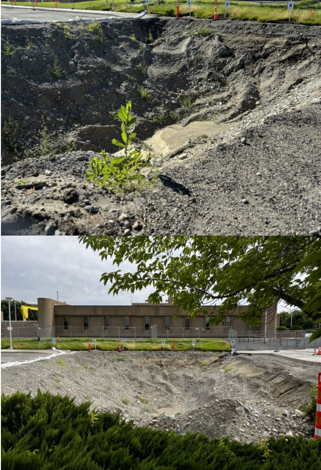
Figure 12. Recent photos (July 2024) of the site show evidence of runoff entering the Tank Pit and fine sediments deposited in the bottom.
