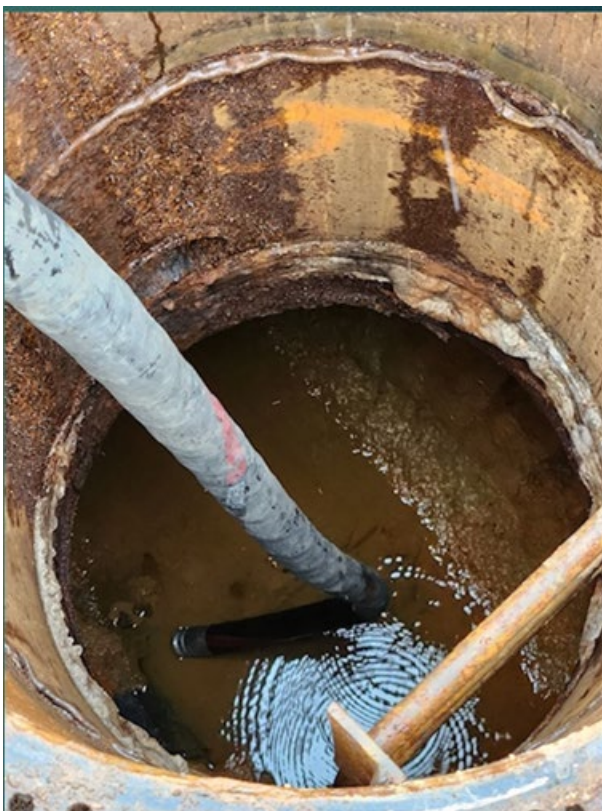
Figure 5. Water is being removed from the tank prior to excavation.
