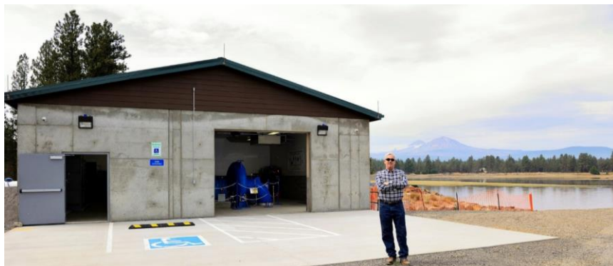
Figure 12. Marc Thalacker, former manager of the Three Sisters Irrigation District in Central Oregon, stands in front of the district's 700 kW Watson Hydropower Facility after installation in 2014. (Photo Credit: Energy Trust of Oregon)
