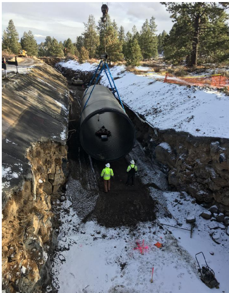
Figure 7. Large diameter pipe installation. (Photo credit: Central Oregon Irrigation District)
