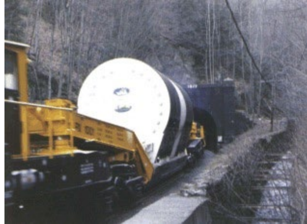
Figure 3-15: Removal of YR Pressure Vessel
