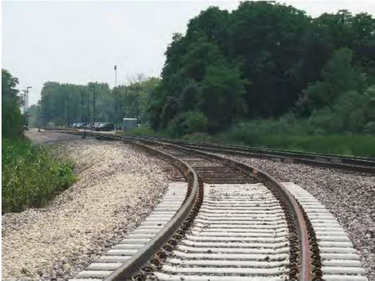
Figure 2-15: Junction of Zion On-Site Rail Spur with Union Pacific Railroad Showing Concrete Rail Ties (2013) [6]
