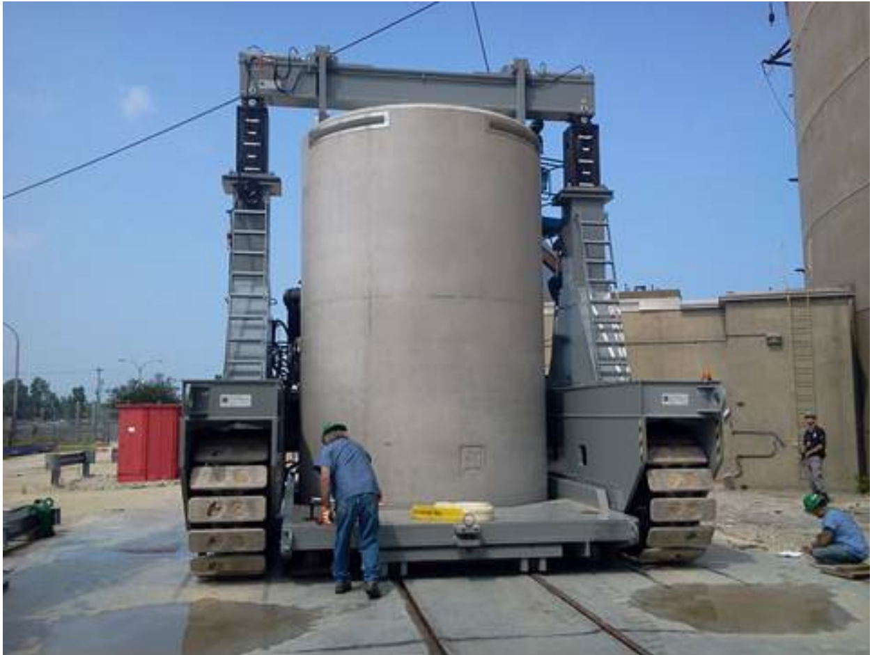
Figure 2-17: MAGNASTOR Vertical Zion VCC Engaged to VCT and Being Removed from LPRC
