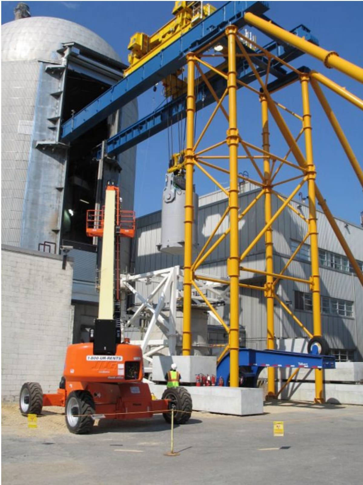
Figure 2-30: MPC-LACBWR TFR Moving to Transfer Position on VCC and TFR Restraint System
