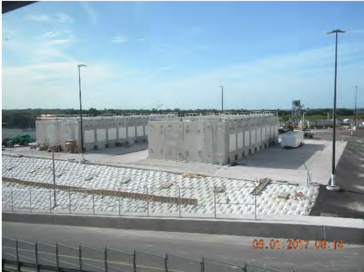
Figure 2-6: Crystal River Independent Spent Fuel Storage Installation with Horizontal Storage Modules Installed [2]
